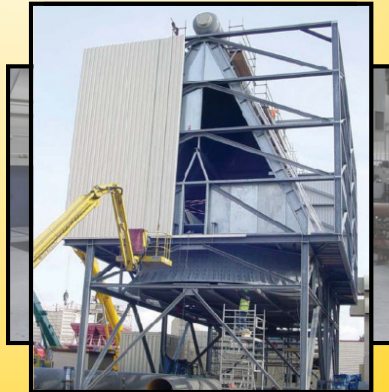
Linear Fresnel Collector, Solar Power Group
